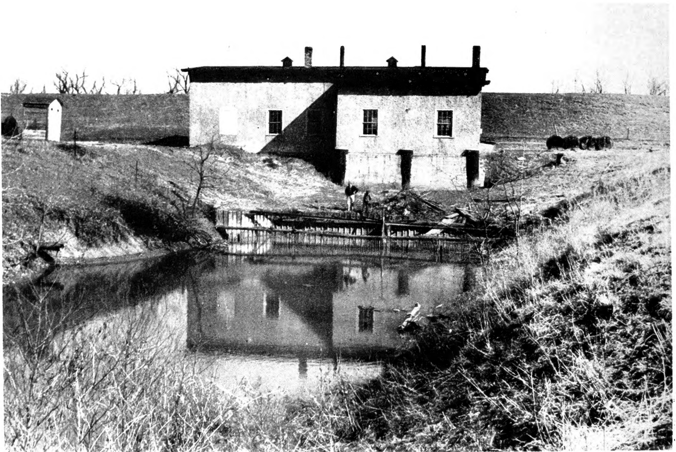
Fig. 2.--Pumping station of levee district bordering the Illinois River. Levee shown in fig. 1 is in background. Surplus water is pumped into the river on the other side of levee to prevent inundation of drained lake basin by seepage or precipitation.
